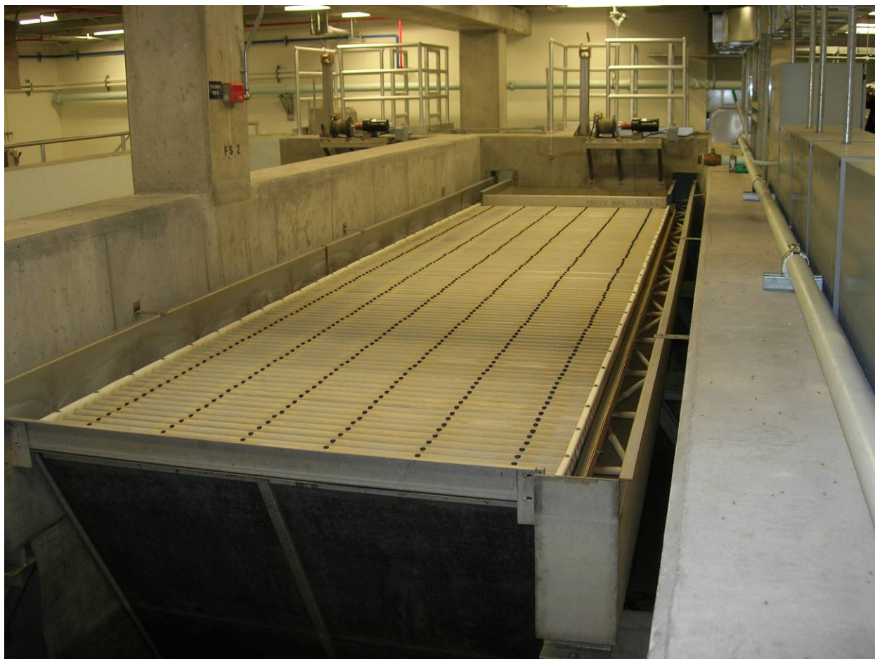
Empty rectangular clarifier with inclined plate settlers at Snake River WWTTP
